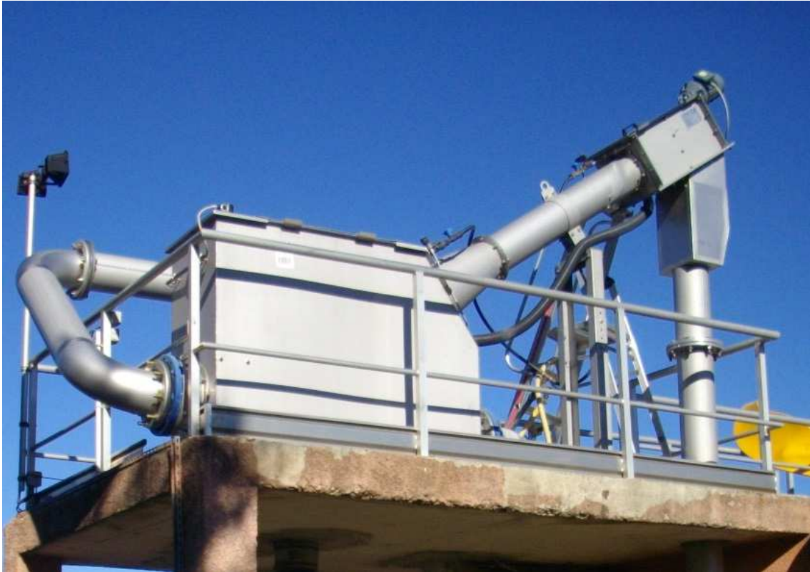
Figure 9 - CFT-C screw screen compactor in tank
