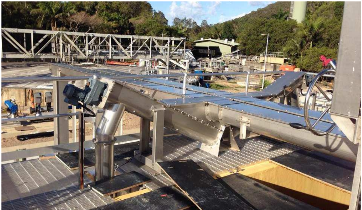
Figure 30 - CCS shaftless screw conveyor in plant with rock trap
