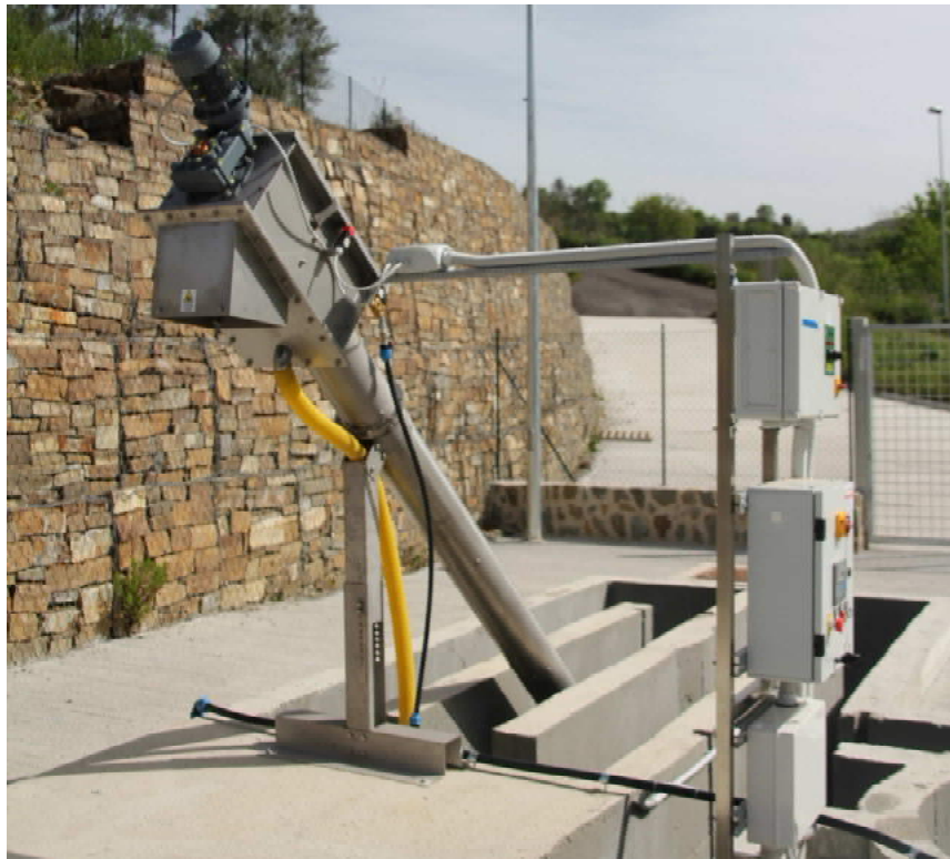
Figure 11 - CFC screw screen compactor in channel
