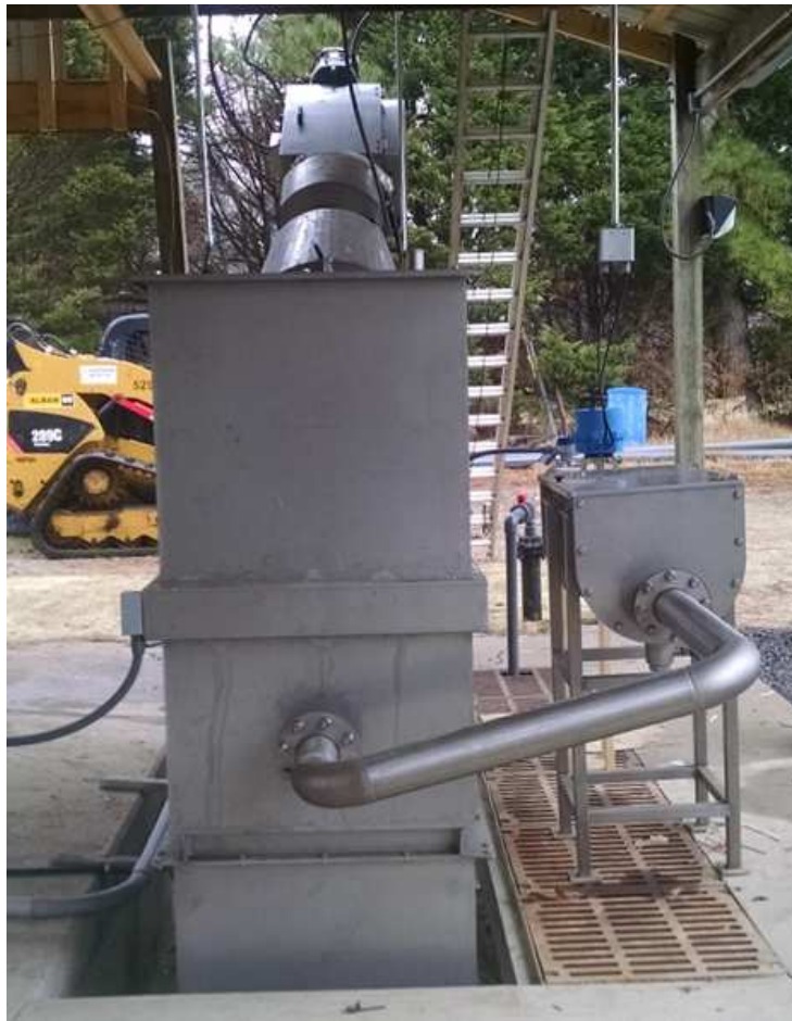
Figure 51 - SAU1 single function septic pretreatment unit in plant
