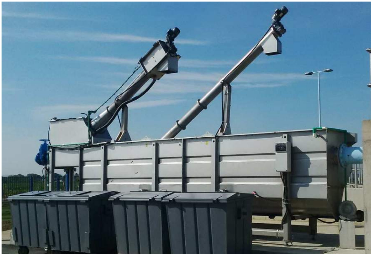
Figure 46 - WAU3 combined pretreatment unit in plant
