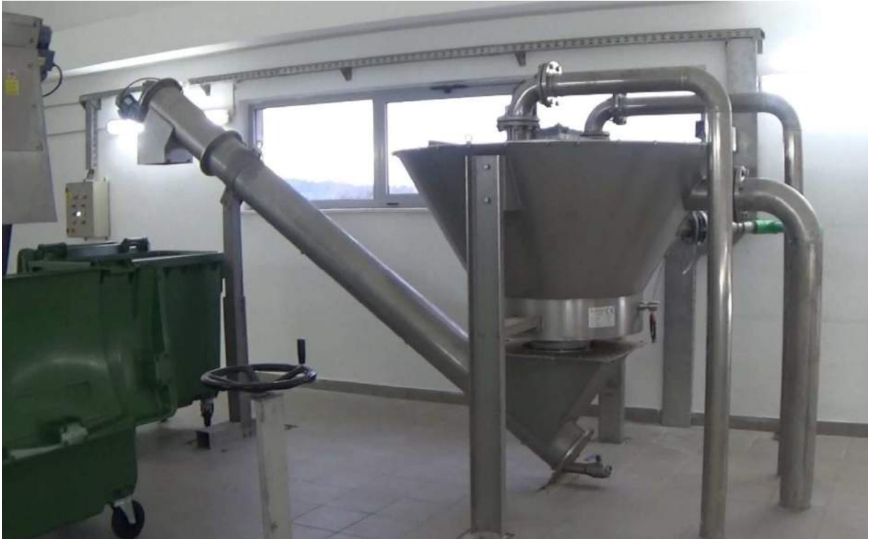
Figure 43 - CDL grit washer in plant
