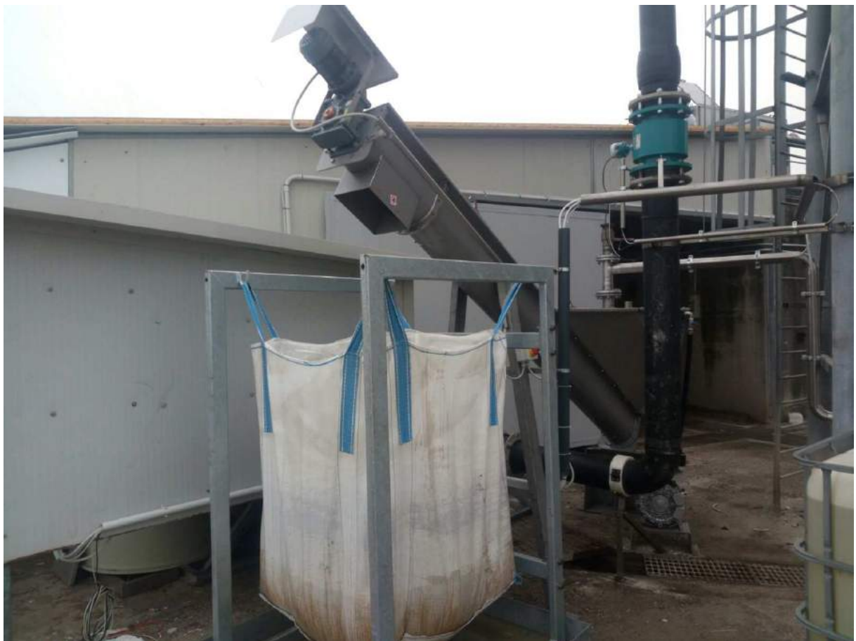
Figure 42 - CDS grit classifier in plant
