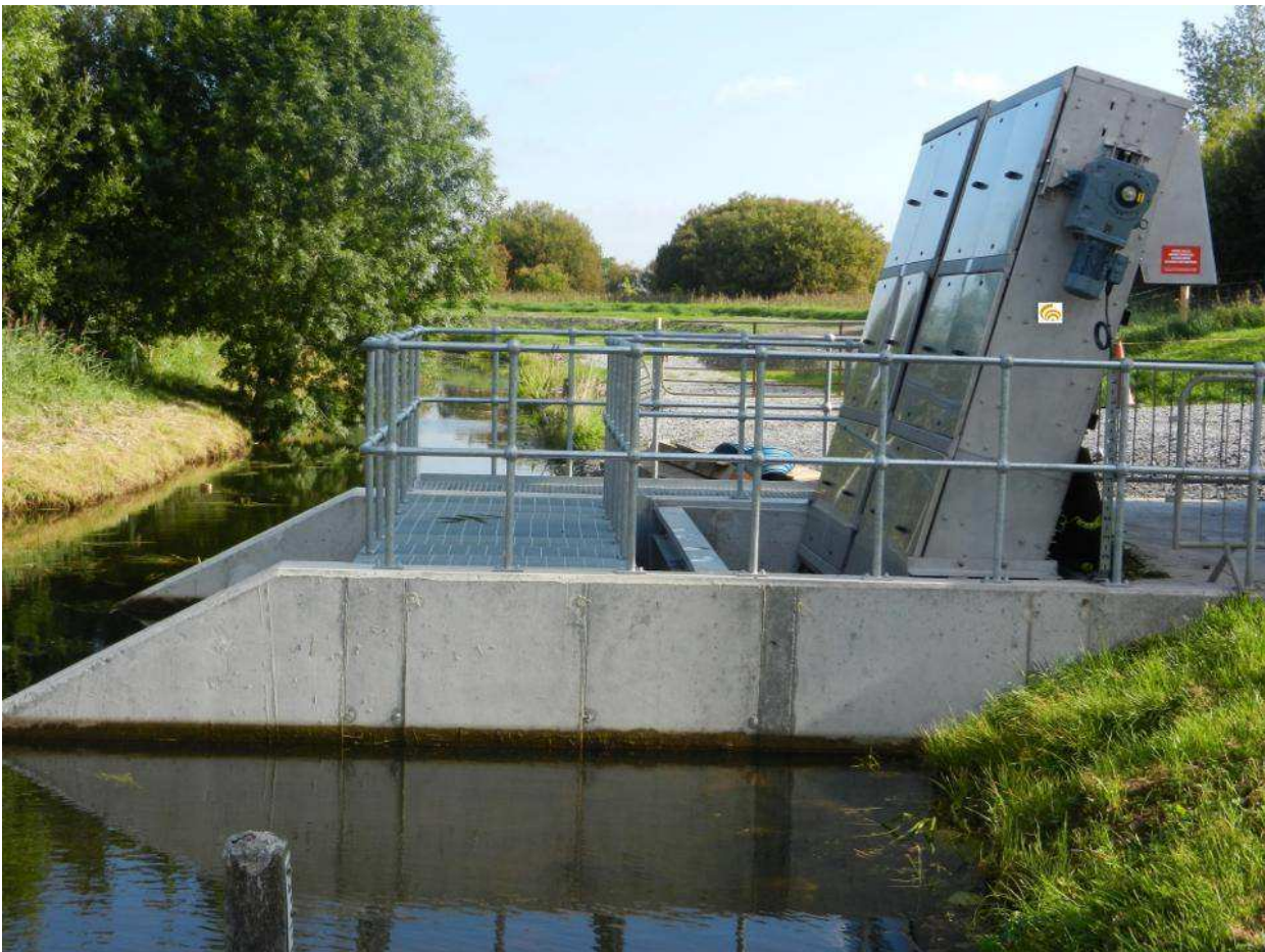
Figure 2 - SMC multi raked bar screen in channel
