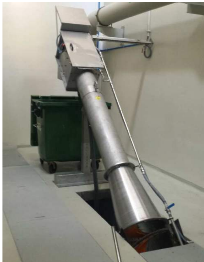
Figure 10 - CFC screw screen compactor in channel
