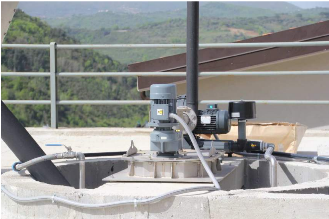
Figure 40 - VXGR vortex grit separator in plant
