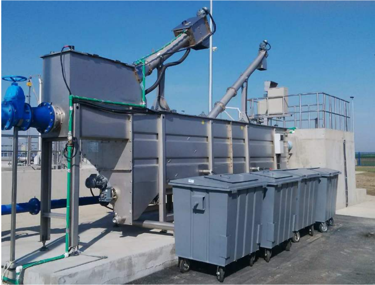
Figure 45 - WAU3 combined pretreatment unit in plant
