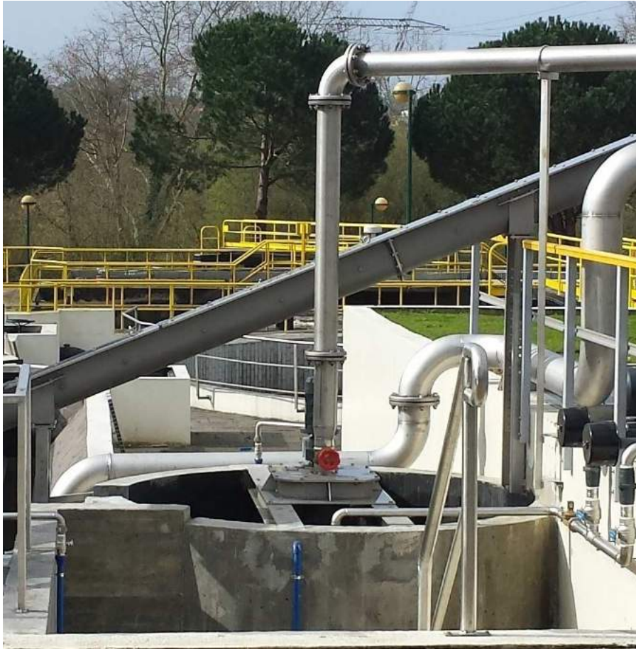
Figure 39 - VXGR vortex grit separator in plant
