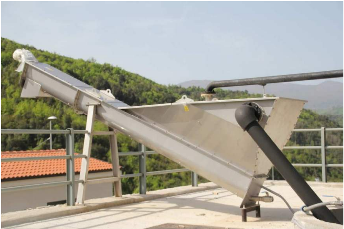
Figure 41 - CDS grit classifier in plant
