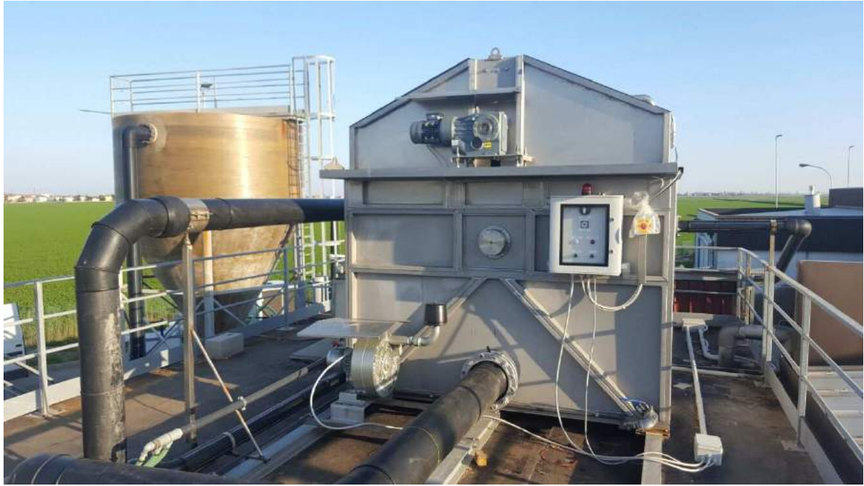
Figure 23 - DFH disk filter
