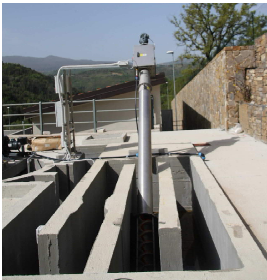
Figure 12 - CFC screw screen compactor in channel
